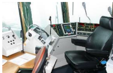
Data processing cabinet for optical landing system
